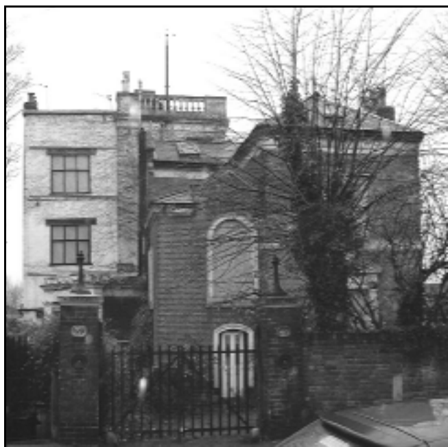
29 LEIGH ROAD TODAY, AWAITING CONVERSION TO 9 FLATS. FORMERLY KNOWN AS BELFIORE LODGE AND AS
