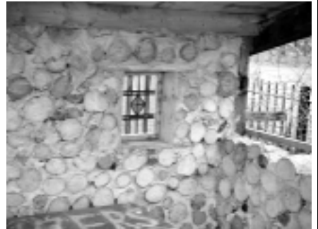
The interior of the Cordwood Hut showing the ends of the logs
