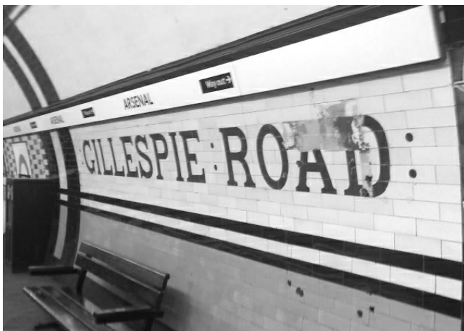
BEFORE (ORIGINAL TILING)
