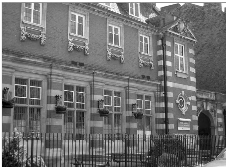
NORTH LIBRARY, MANOR GARDENS
